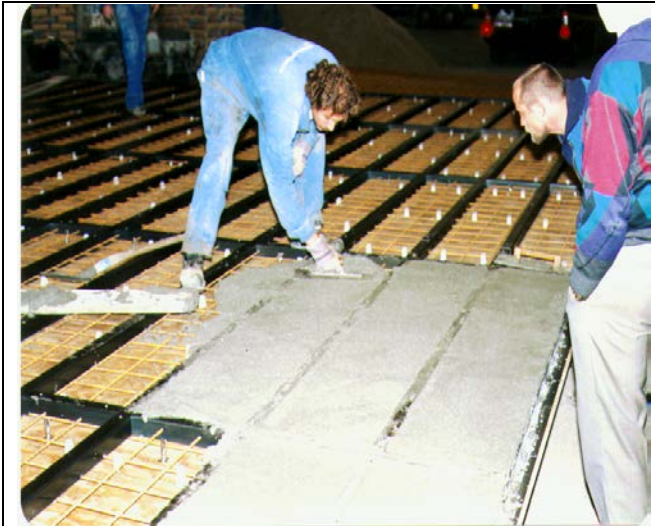
Pre-Fabricated Ceiling Panels Pre-Production tests of LightCem LITECRETE panels were carried out before full scale production and delivery.
