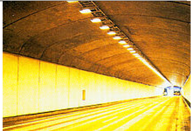
Gothenberg Tunnel – Roof Lining Segments Pre-cast LightCem LITECRETE concrete segments provide the strength without the weight – and therefore reduced costs!
